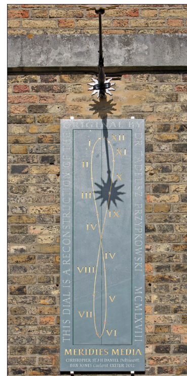
Fig. 1. A vertical mean time noon mark ( mérienne ) at the Royal Observatory at Greenwich. This kind of sundial shows not only the true solar noon (vertical line) but also the mean noon (that is, true noon with the ET correction). When sunlight passing through the eyelet falls upon the analemma curve, local mean noon is easily read as a function of the date (Photograph source: Wikipedia; author: Christopher St J. H. Daniel).
